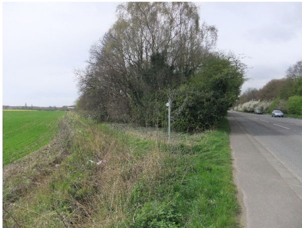
Pavement on southern side of A631 at junction with Public Footpath and required safe crossing point to access the eastern end of Swinnow Wood.
