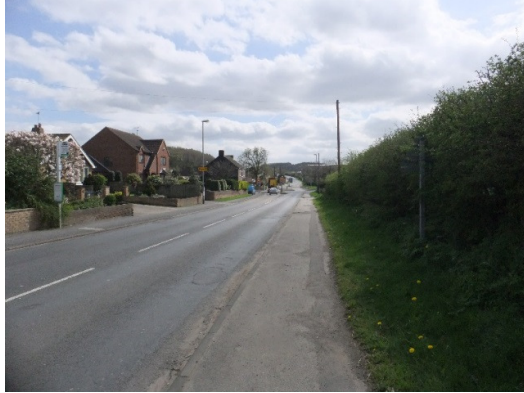
Tickhill Road pavement and grass verge, looking south
